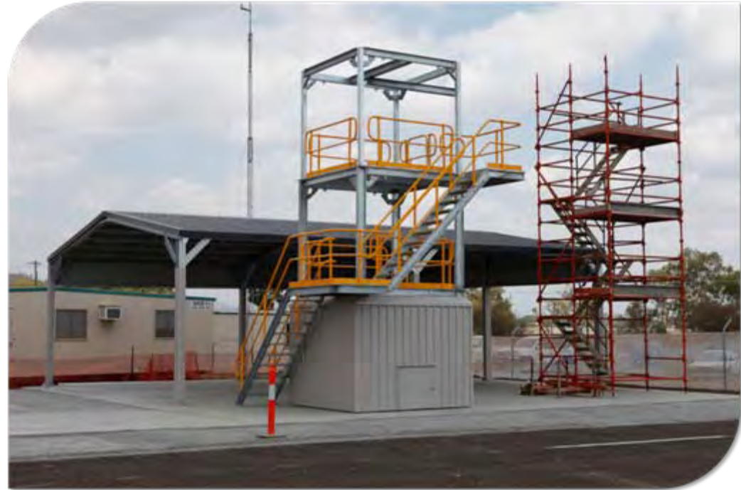
Practical Induction Training Facility
