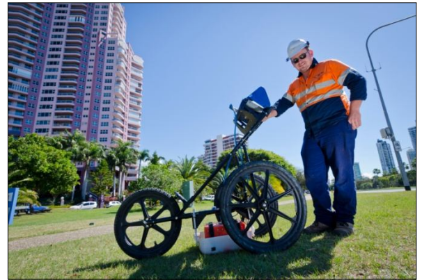
A surveyor with ground penetrating radar unit. Image courtesy of Gold Coast Rapid Transit project
