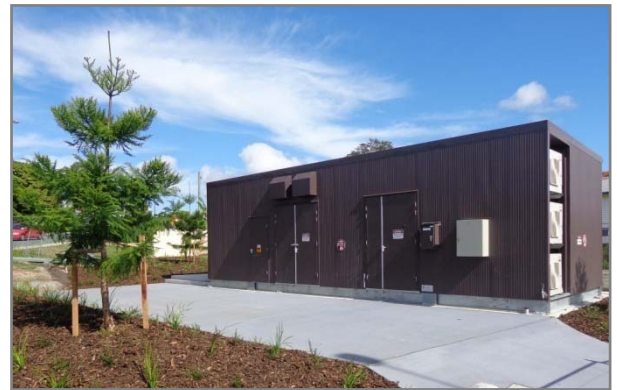
Traction Power Substation
