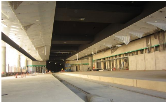
The underground station at the Gold Coast University Hospital
