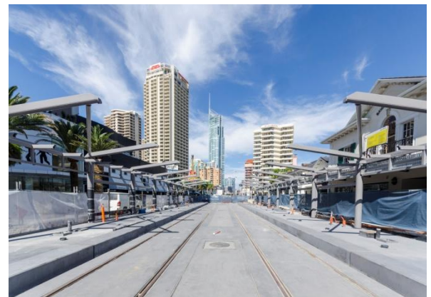
Cavill Avenue Station construction
