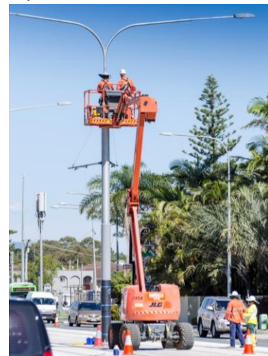
Overhead pole works
