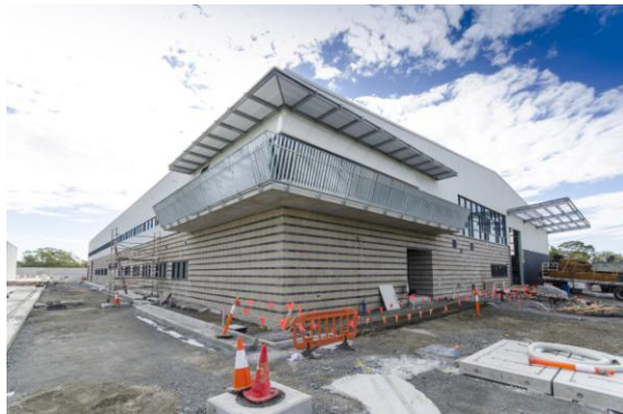
Depot building nearing completion
