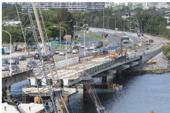
Light rail bridge across the Nerang River
