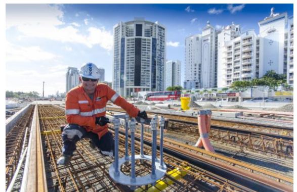
Works installing rail at Broadbeach
