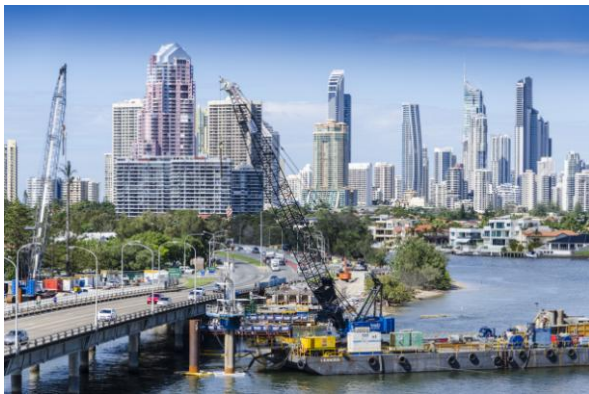
Two barges working on the Nerang River light rail bridge
