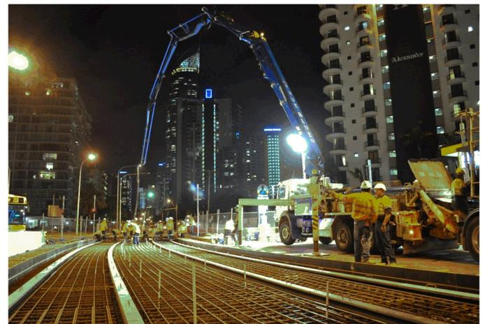
Concrete pump with extended boom. used to pour concrete for rail.
