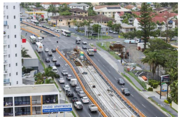
Track work on Gold Coast Highway
