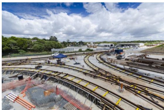
Track laying at the Depot site
