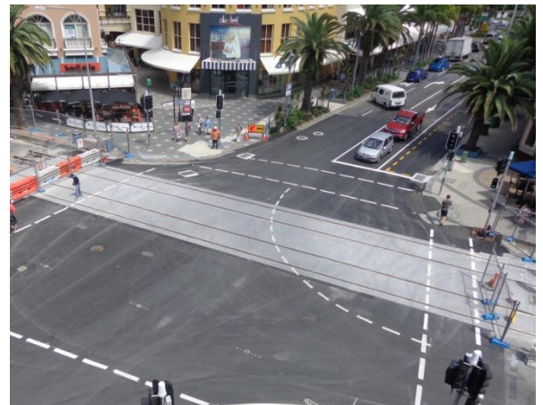
First track installed in Surfers Paradise at Surfers Paradise Boulevard and Elkhorn Avenue intersection
