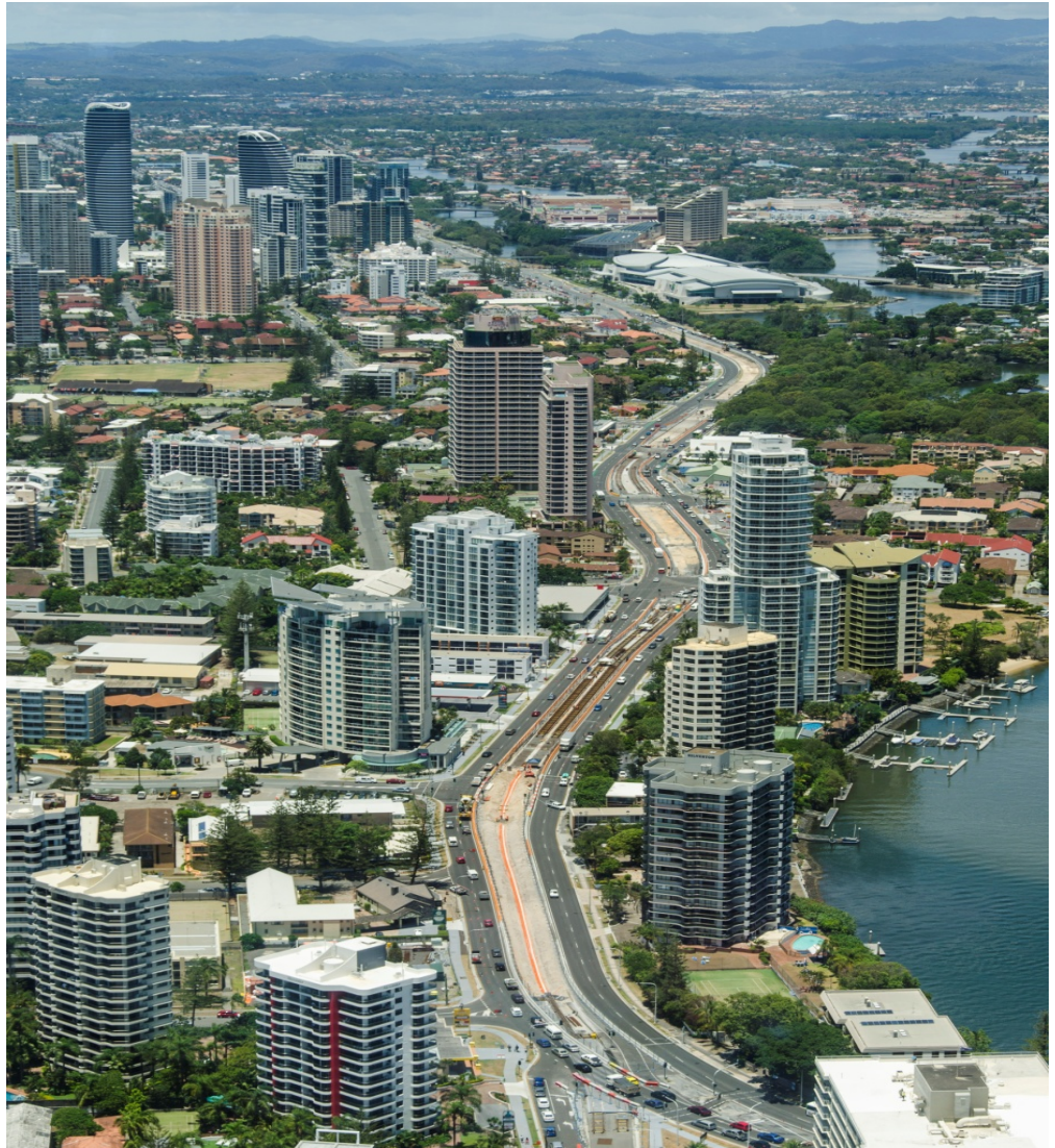
Light rail corridor Gold Coast Highway
