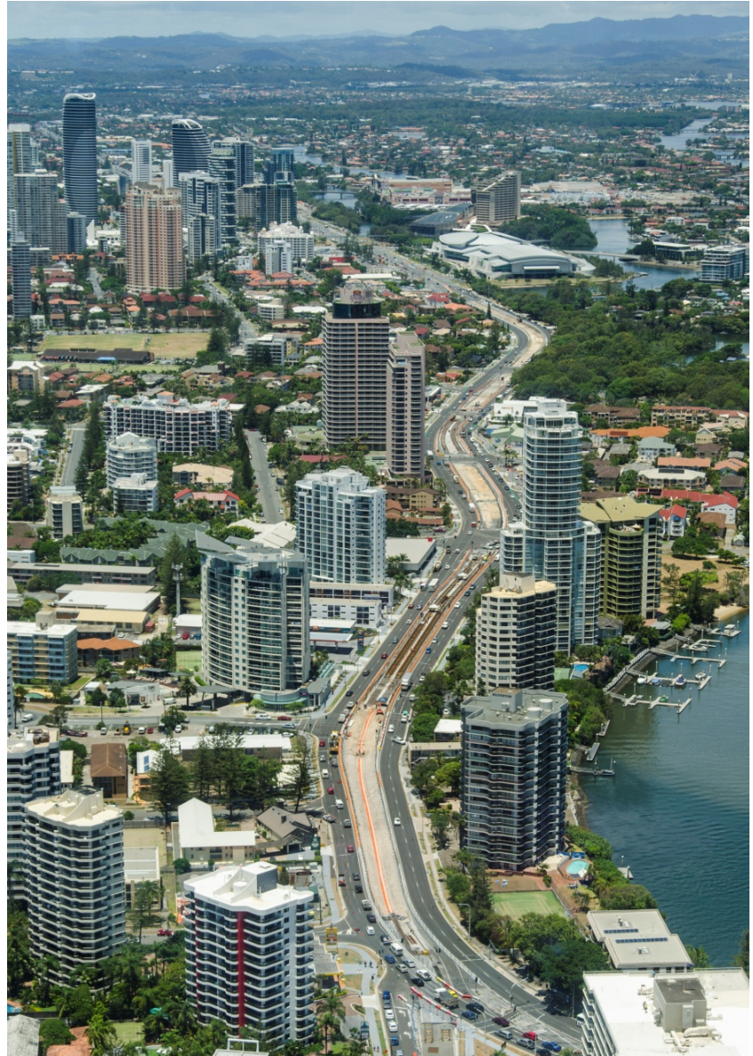
Light rail corridor Gold Coast Highway
